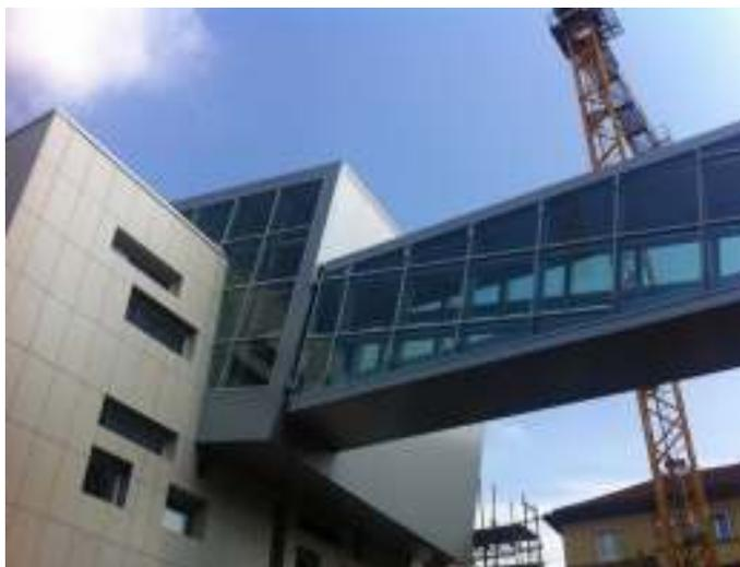
*Designed as a "near-zero energy building", the new headquarters office is an example of installation-integrated building-system. The high insulated envelope, the sunscreens for windows, the absence of thermal bridges, the reduction of air losses and the use of a heat recovery unit with an efficiency of over 80%, ensure maximum comfort inside the workplace.*
